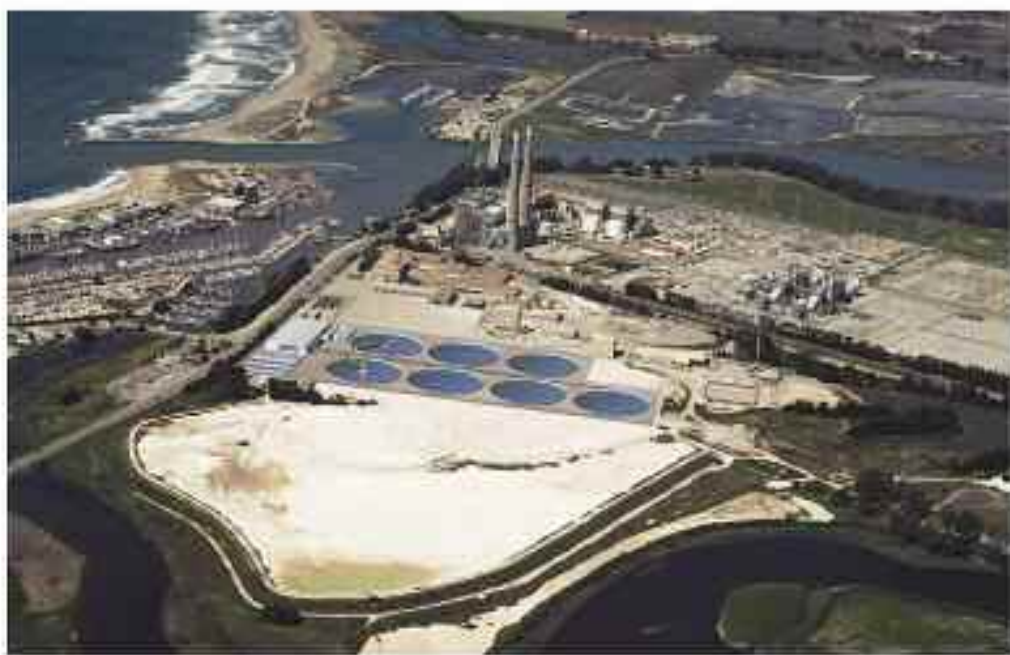
Proposed Moss Landing Desal facility
